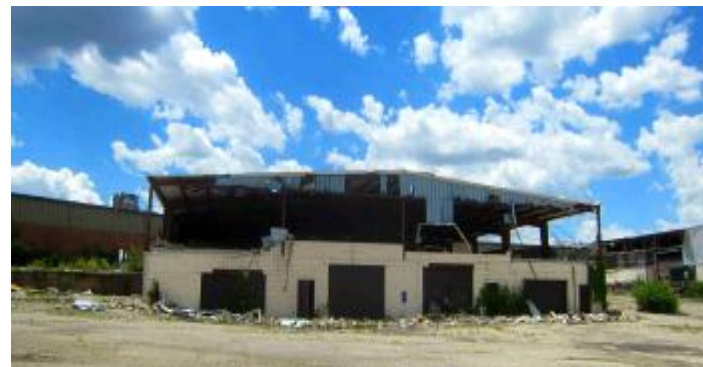
The rear of the Ball Arena had concrete block walls blown out and the concession area roof collapsed. I guess all this has sealed the fate of the old girl, but, I just had to stop by and take one last look at our old Hamvention haunt.
