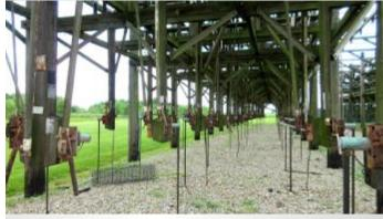
The switchyard contained dozens of high voltage switches directing the RF into selected antenna arrays. When time came for a band change, the transmitters were turned off and technicians would run out in the yard and set the switches into the proper position. The Chief Engineer would stand at
